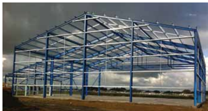
Stage 1 Paint facility under construction
